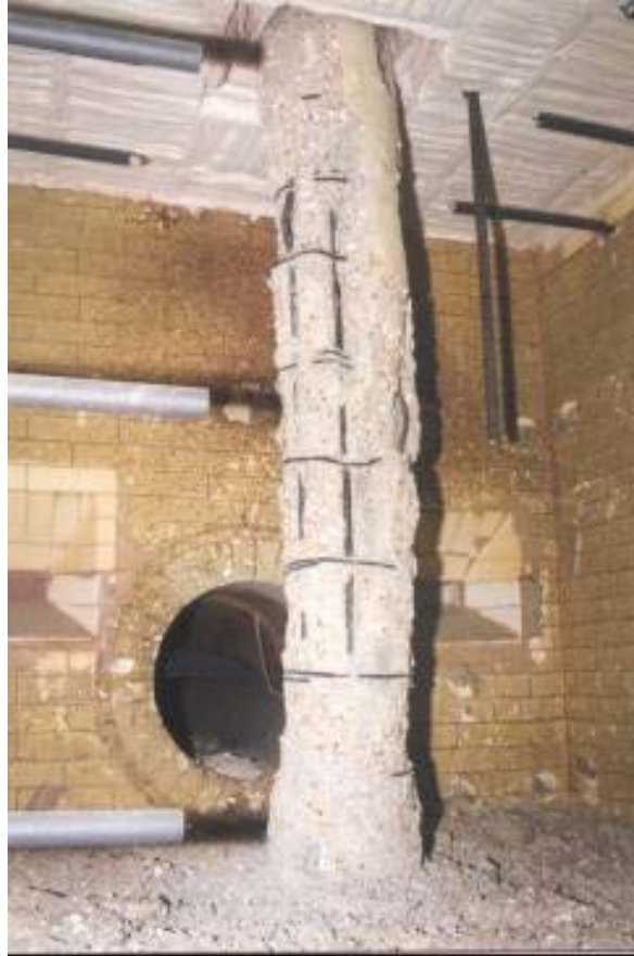
Fig. 4: spalling in column C1 as observed after the test
